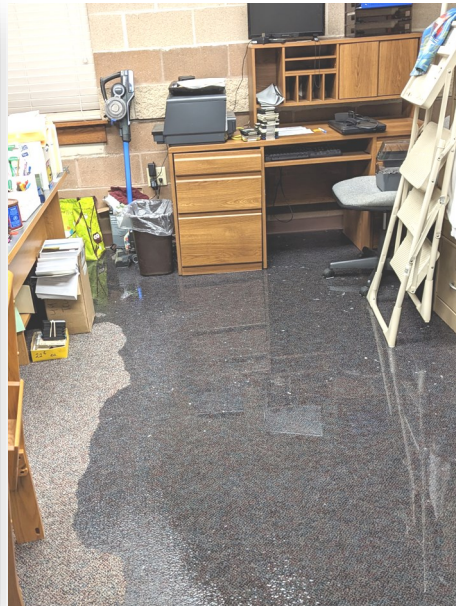
Main Hall & Offices
